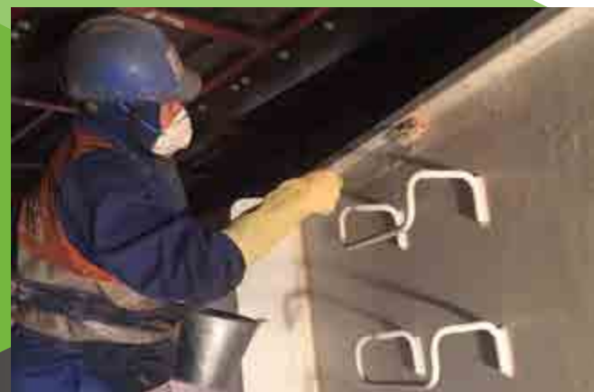
FGD, SCR, Absorber (Flake Lining) Blasting and painting Ceilcote Ha Tinh Formosa Project
