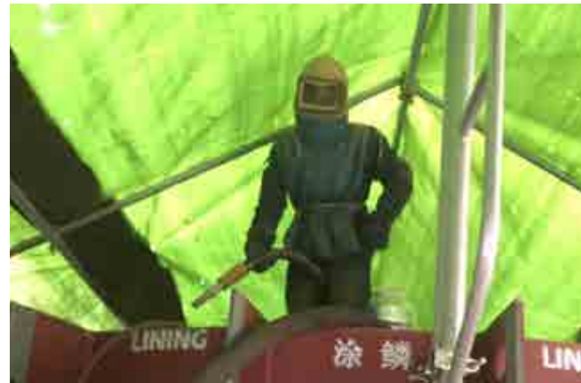
FGD, SCR, Absorber (Flake Lining) Blasting and painting Ceilcote Ha Tinh Formosa Project
