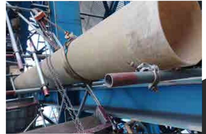
Fabrication & Installation Ash Chute U1, 2 Mong Duong 2 Thermal Power Plant
