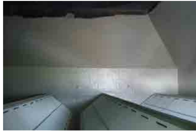
FGD Blasting & Painting - Ceilcote (Flake Lining) NSRP Project
