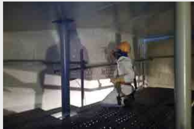
FGD Blasting & Painting - Ceilcote (Flake Lining) NSRP Project
