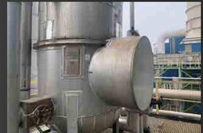
Insulation Installation (TA) AmonNitrat Thai Binh
