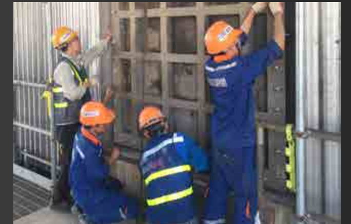
Absorber heat exchangers Replacement Mong Duong 2 Thermal Power Plant
