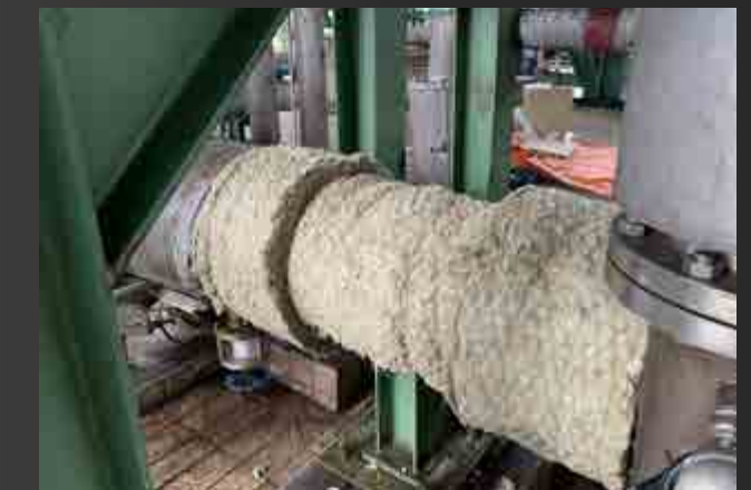
Insulation Installation (TA) AmonNitrat Thai Binh
