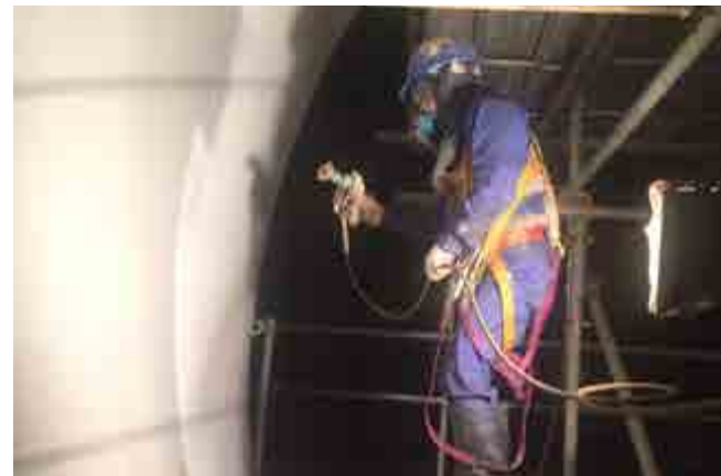
FGD, SCR, Absorber (Flake Lining) Blasting and painting Ceilcote Ha Tinh Formosa Project
