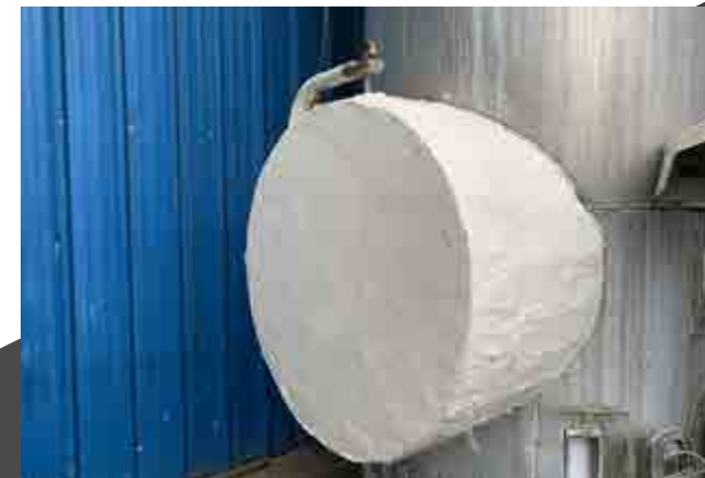
Insulation Installation (TA) AmonNitrat Thai Binh
