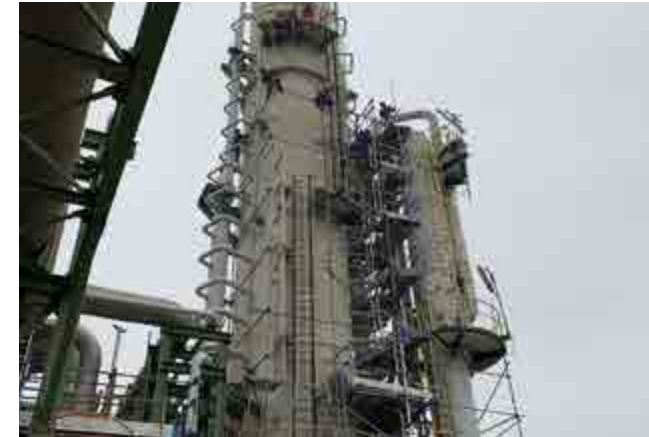
Scaffolding Erection AmonNitrat Thai Binh
