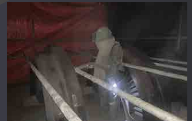
Turbine Equipment Blasting Vung Ang 1 Thermal Power Plant
