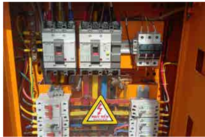
Socket Panel for ESP&SDCC Install Service Mong Duong 2 Thermal Power Plant
