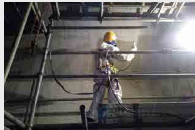
FGD Blasting & Painting - Ceilcote (Flake Lining) NSRP Project
