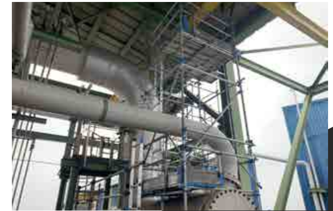
Scaffolding Erection AmonNitrat Thai Binh
