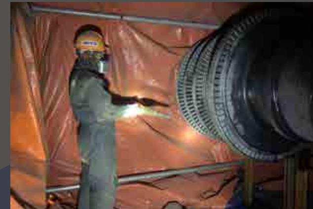
Turbine Equipment Blasting Vung Ang 1 Thermal Power Plant
