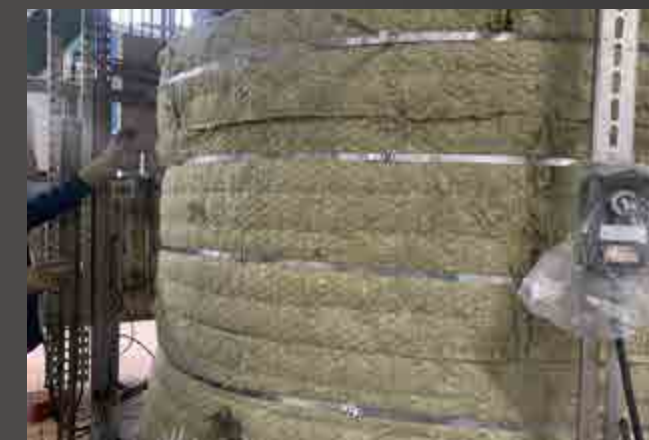
Insulation Installation (TA) AmonNitrat Thai Binh
