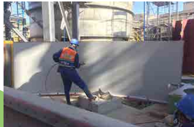
FGD, SCR, Absorber (Flake Lining) Blasting and painting Ceilcote Ha Tinh Formosa Project
