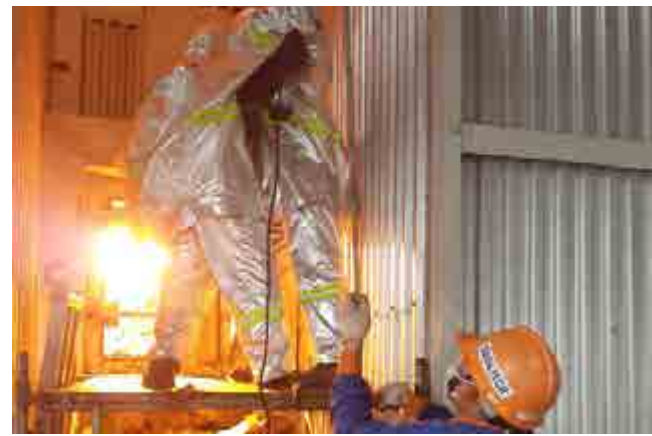
Remove Coal slag Thai Binh 1 Thermal Power Plant
