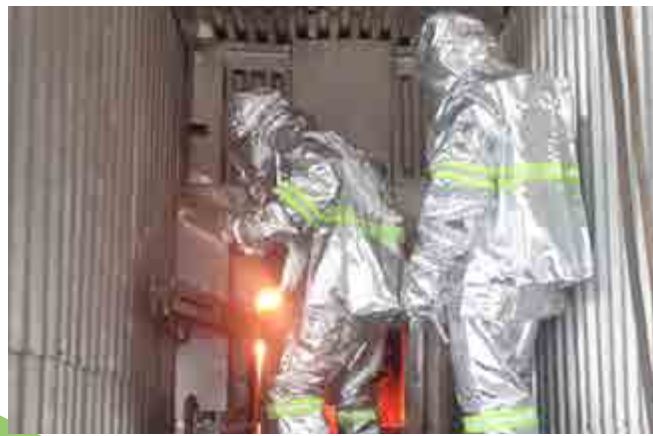
Remove Coal slag Thai Binh 1 Thermal Power Plant
