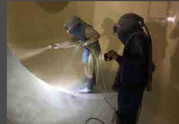
Blasting and Painting CWP (Polibrid) Mong Duong 2 Thermal Power Plant
