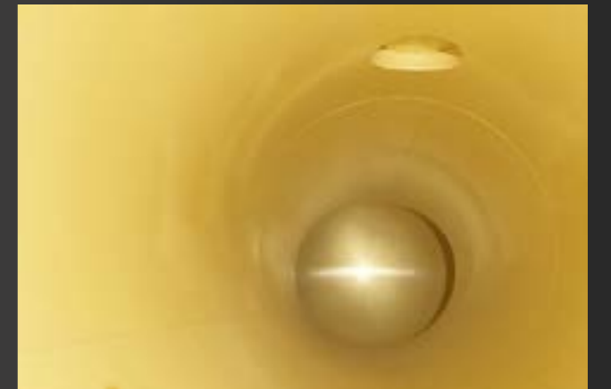
Blasting and Painting CWP (Polibrid) Mong Duong 2 Thermal Power Plant
